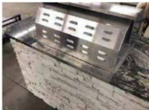
View behind the island after Grill Head is placed
